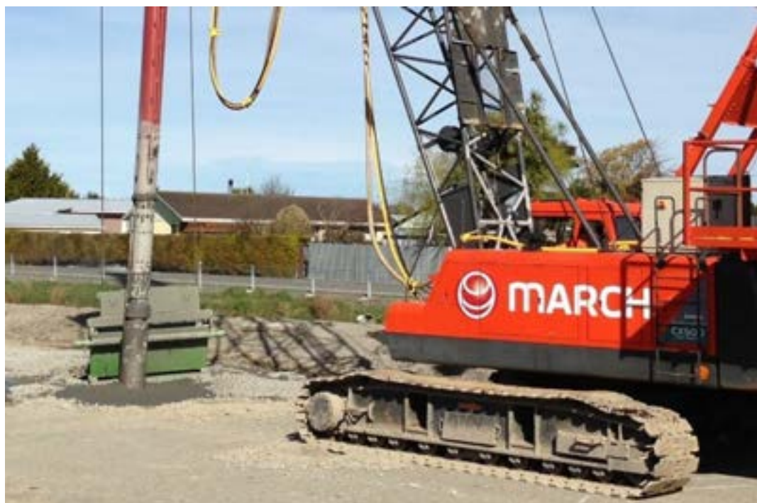
Fig A2. Well compacted granular platform
