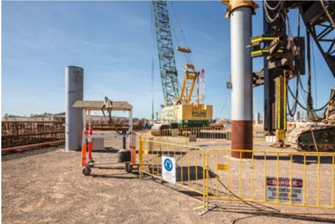
Fig A1. Good demarcation of piling activities
