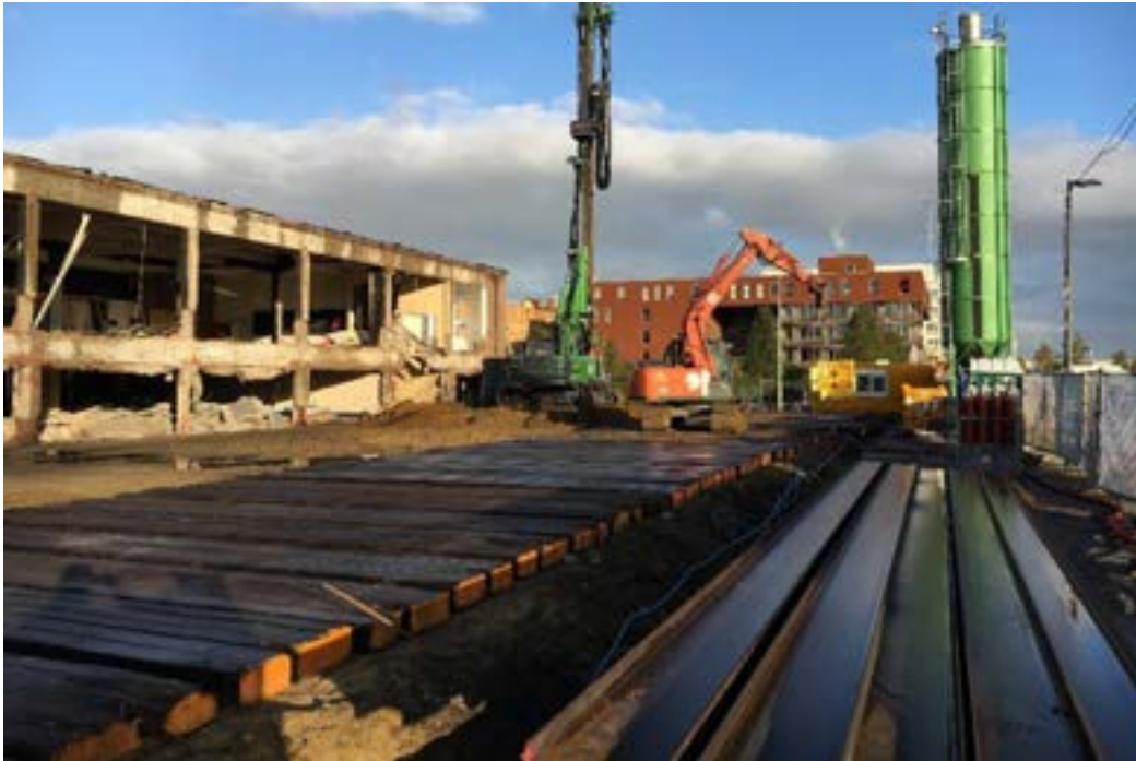
Fig A9. Use of timber mats to form a working platform
