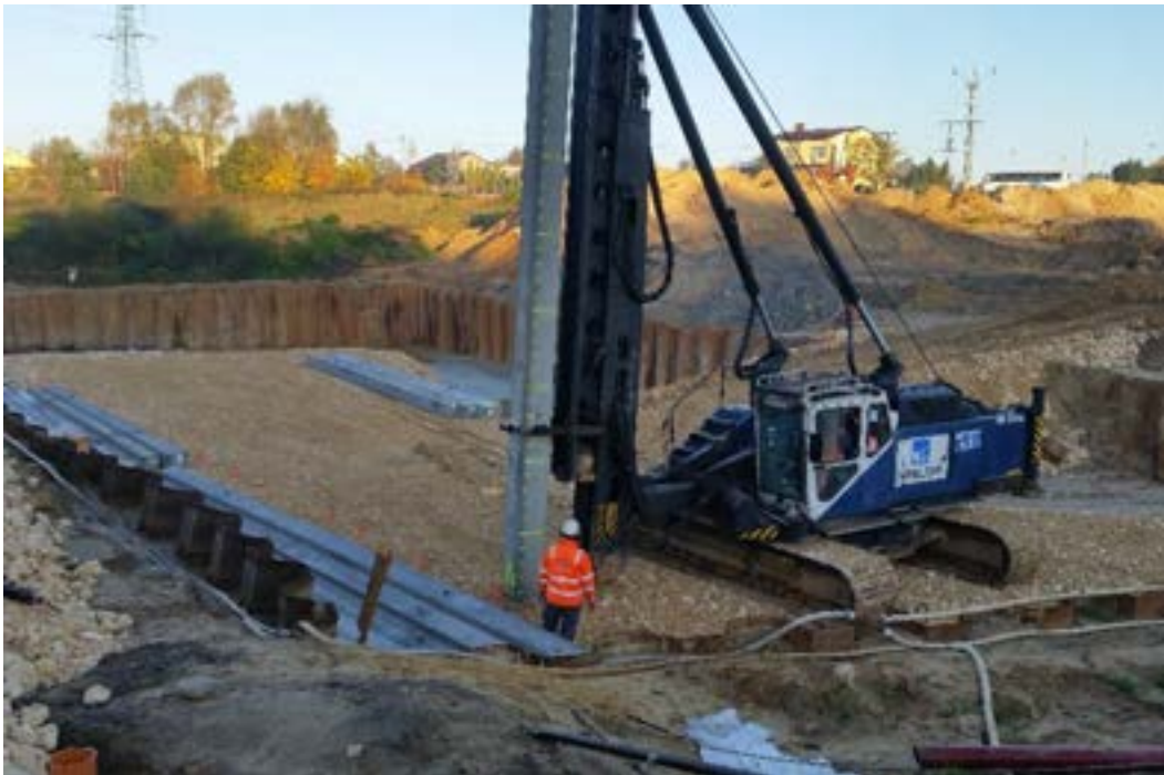
Fig A5. Example of a platform with dewatering
