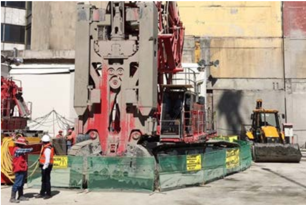
Fig A3. Example of a concreted platform
